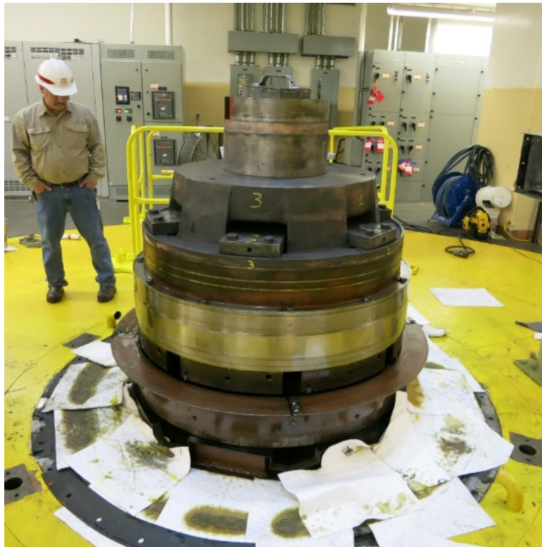
Figure 13. Unit 2 Disassembled Showing the Combination Generator Thrust Bearing/Upper Guide Bearing
