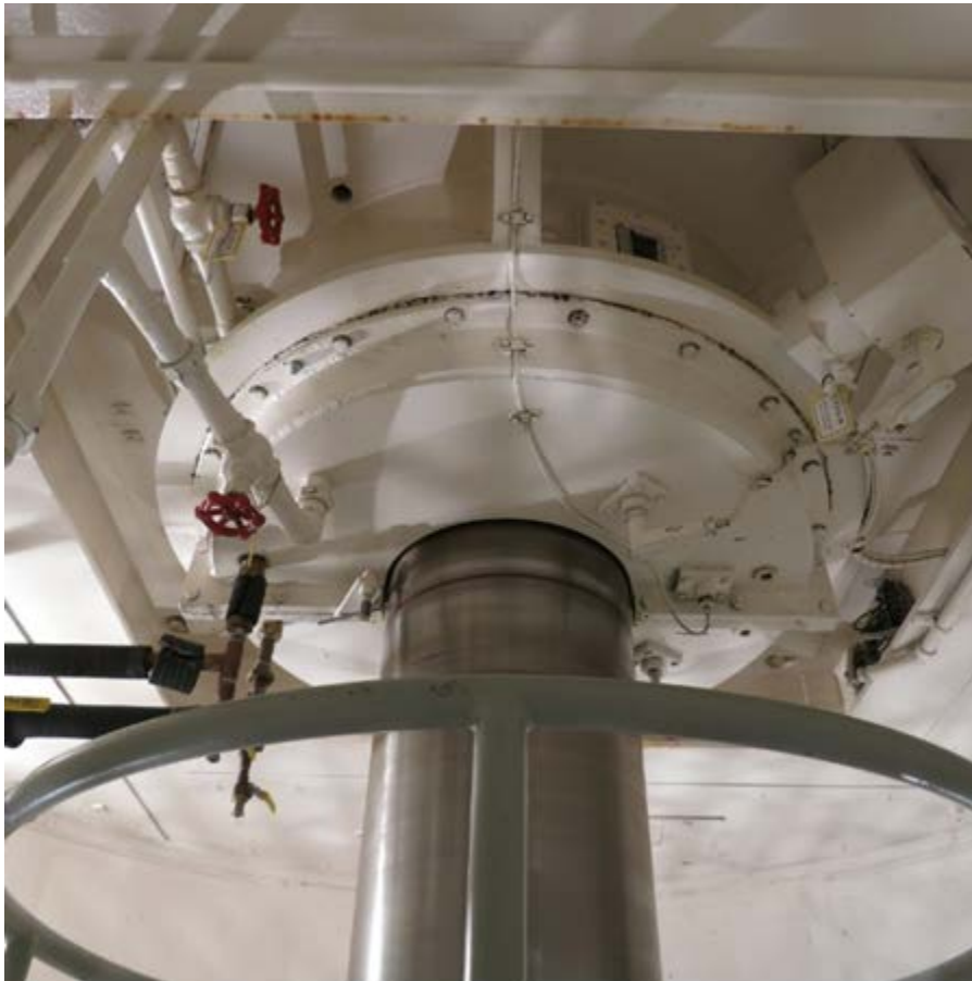
Figure 14. Lower Generator Guide Bearing
