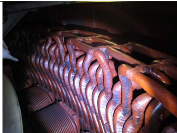
Photo B. Unit 1 Upper End-Windings and Connections
