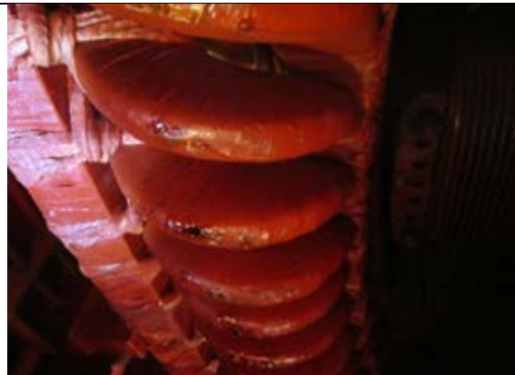
Photo D. Unit 2 Lower End-windings
