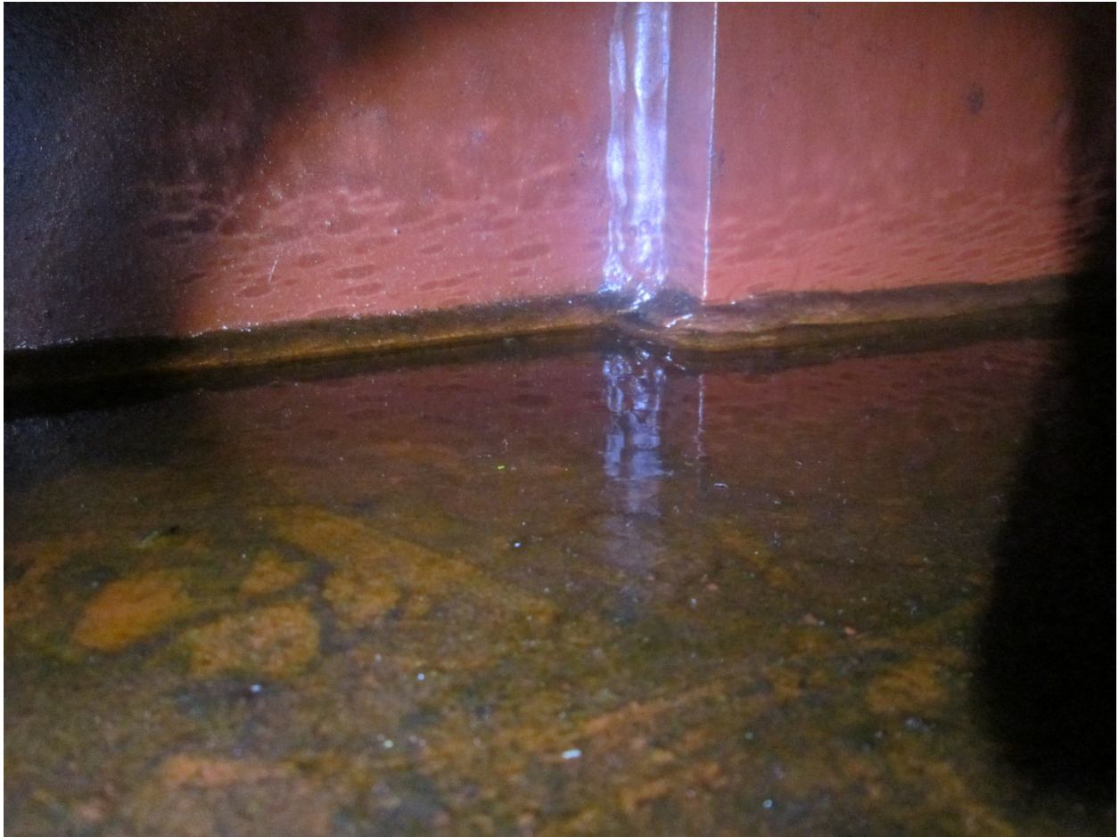
Photo G. Oil Found on the bottom of Unit 2 Generator Frame
