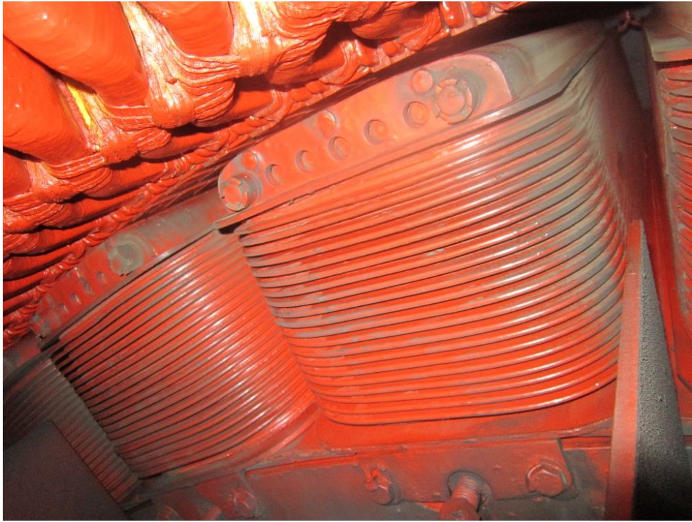
Photo E. Unit 2 Rotor Poles
