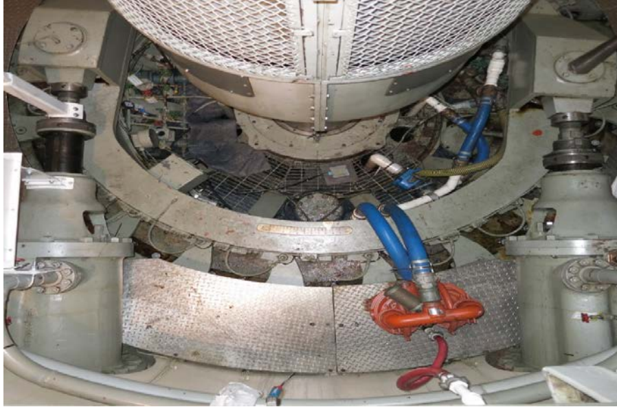
Figure 15. The Turbine Pit Showing the Two Wicket Gate Servos and the Wicket Gate Linkage.
