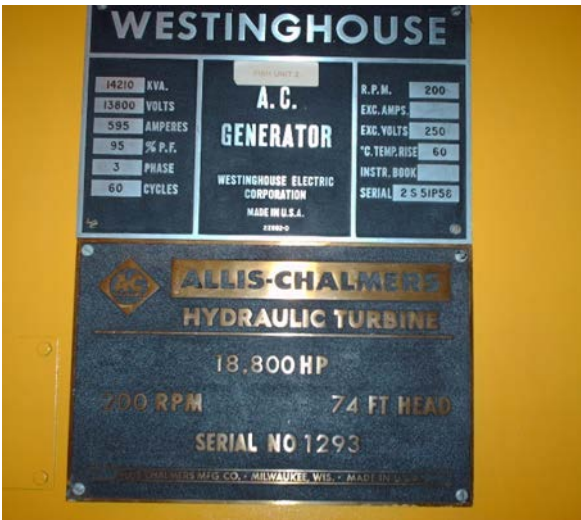
Figure 1. Generator Nameplate
