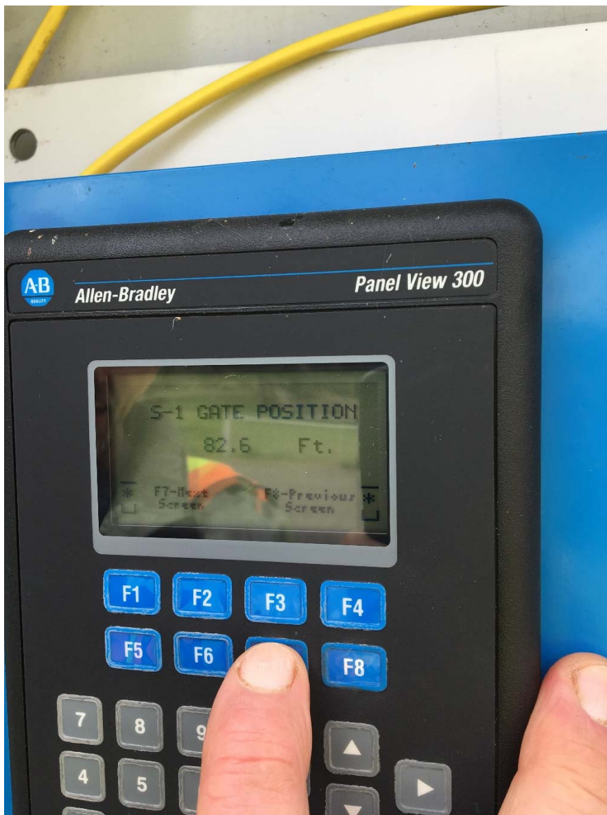
Photo 4: Panel outside of PH showing gate position in EFL entrances, typ.
